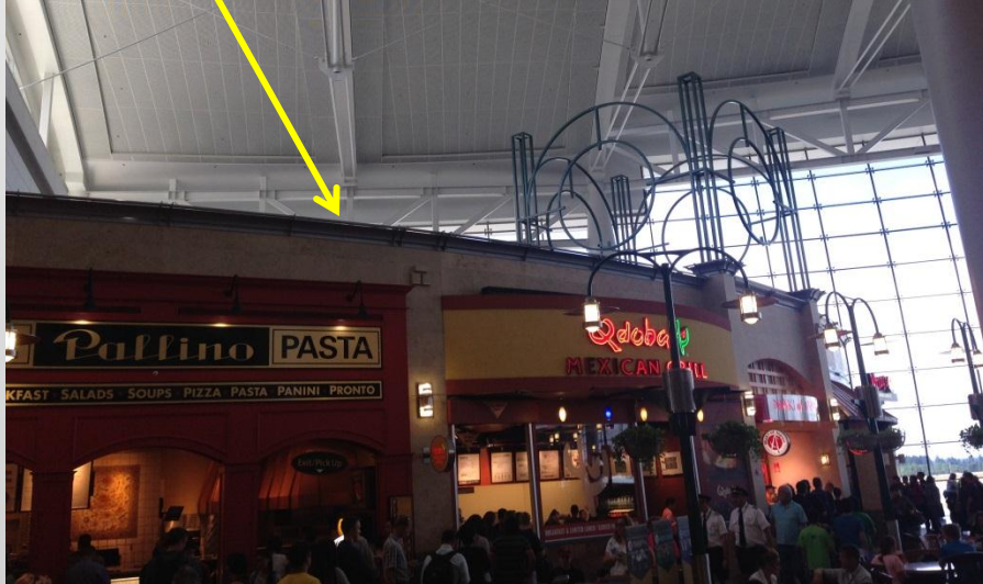
SOUTH MEZZANINE SPACE
